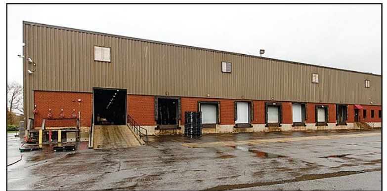
400 Manley Street - Bridgewater, MA
